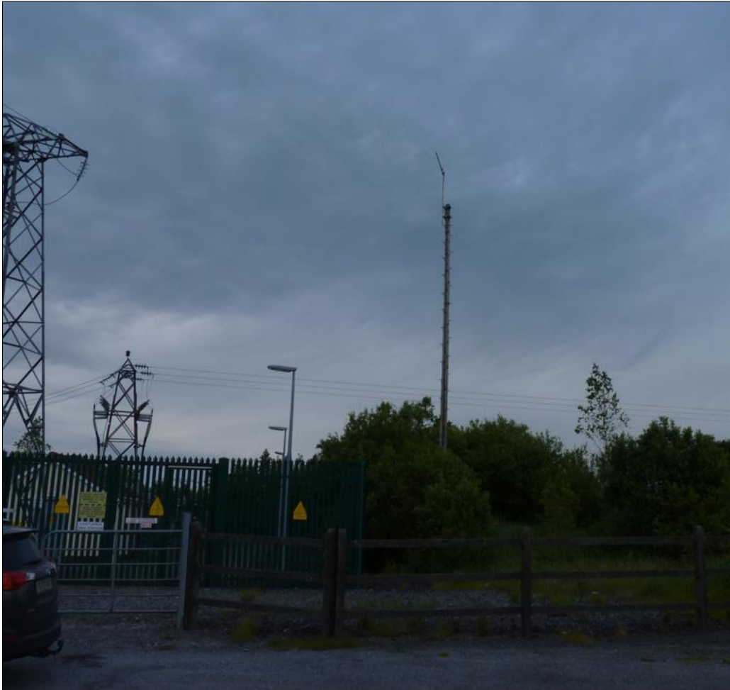
Figure 5. ESB Antenna at Glenamaddy 38kV Station
